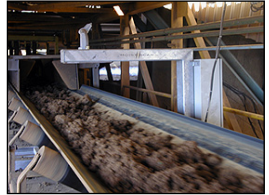
MA-500 installed on conveyor
