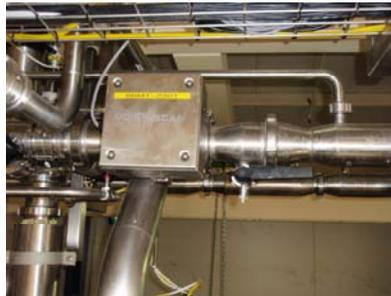
**MA-700 In-pipe analyser on condensed milk line**
